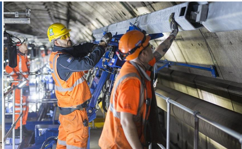
Installation of HEX beams in the North railway tunnel
