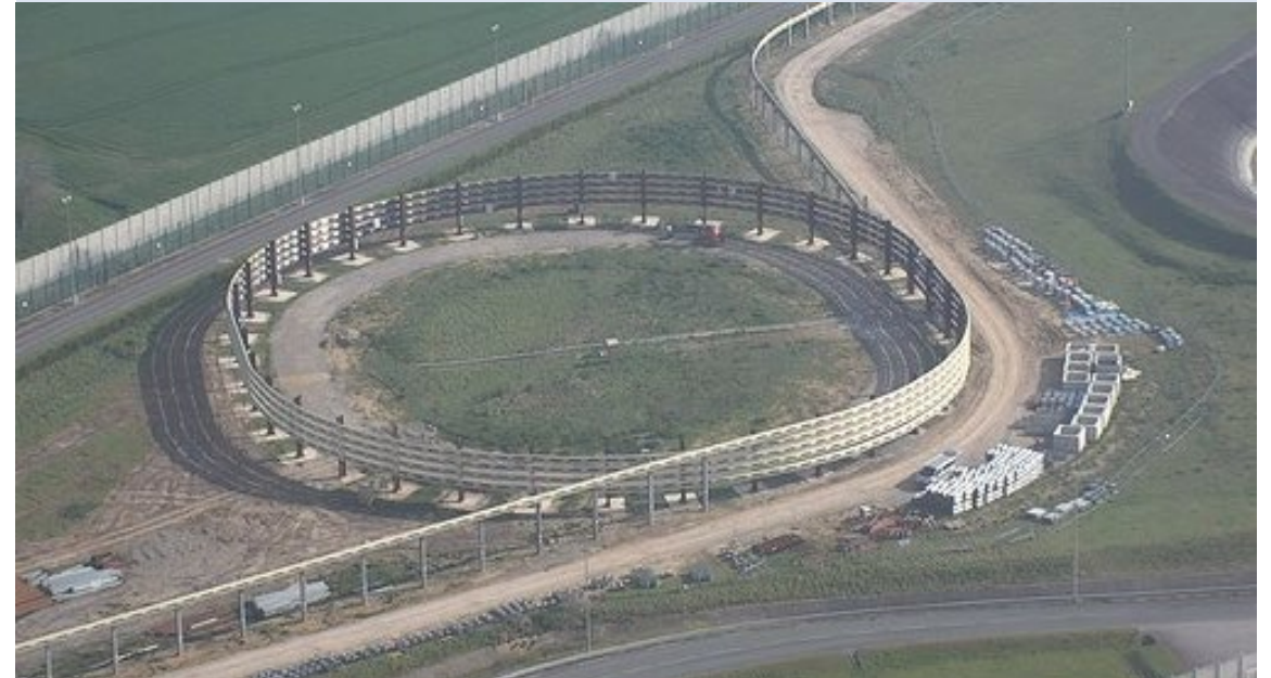
Helix for cable pulling
