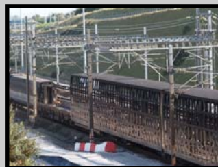
Apart from soot deposits, the loader and the first three wagons appear to be intact.
