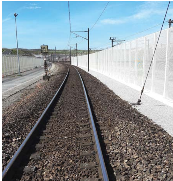
Surrounded by 4m high security fencing and automated gates, the 850-metre long siding track constitutes a secure area if a Truck Shuttle needs to stop.
