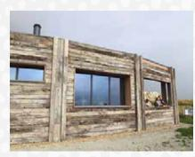
Co-financed by Eurotunnel and the Heritage Lottery Fund, the Education Shelter was built using environmentally friendly construction criteria. It is wood framed and the exterior for the back is clad using recycled railway sleepers from the Eurotunnel terminal in France and larch for the front. The shelter will be heated by wood-fired stoves. Eurotunnel Group has again delivered a benefit to the local community.
