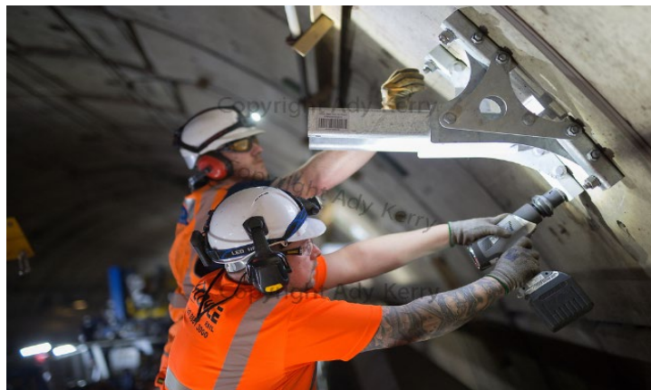
Figure 15: Installation of monorail system in the north running tunnel
