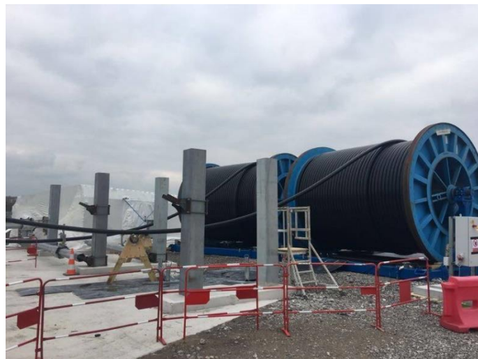
Figure 8: HVDC cable drums
