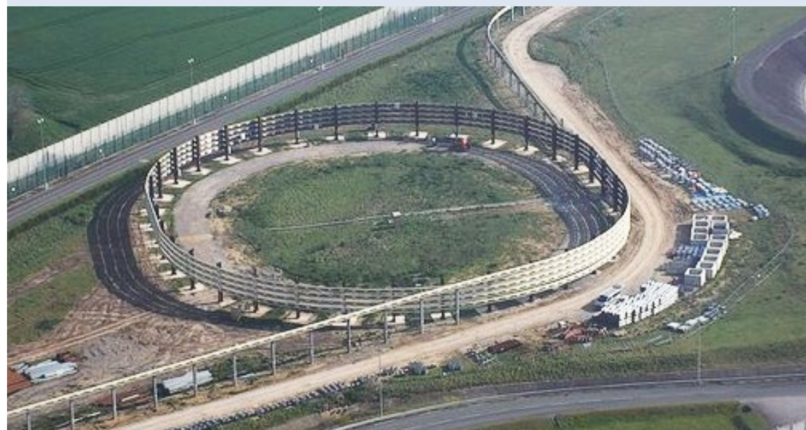
Helix to pull the cable
