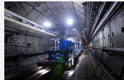
DC Cable hauling in the Tunnel completed in May 2021
