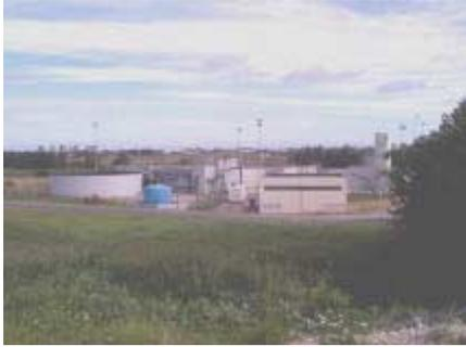
The urban biological purification plant built by Eurotunnel in France, has a design capacity equivalent to a population of 13,500 people. This water treatment plant treats the wastewater from Eurotunnel and from Coquelles.
