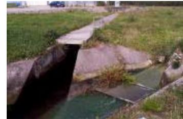
Eurotunnel took this historical local feature into account in the design of the French Terminal: watergangs (drainage ditches) and streams were fitted out after a hydraulic enquiry. The hydraulic systems put in place by Eurotunnel maintain the flows of water on and off the Terminal. The self regulating water quality systems were improved in 2002 on two of the four storage reservoirs designed to allow the control of the discharges and the quality of surface water released to the sea.
