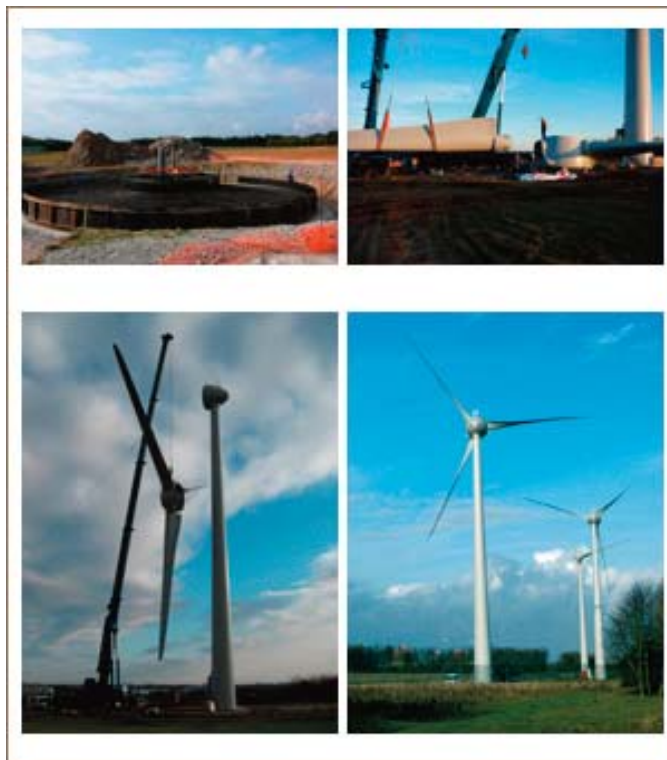
Various stages of the construction process of the 3 turbine wind farm
