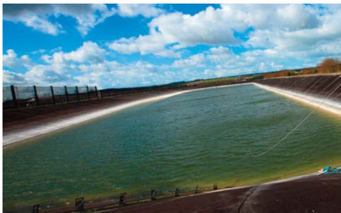
One of the buffer reservoirs on the Coquelles Terminal
