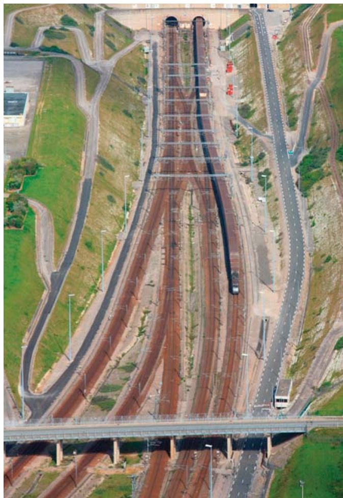
Coming from Folkestone (UK), a Passenger Shuttle exits the Channel Tunnel in the Beussingues trench (FR)
